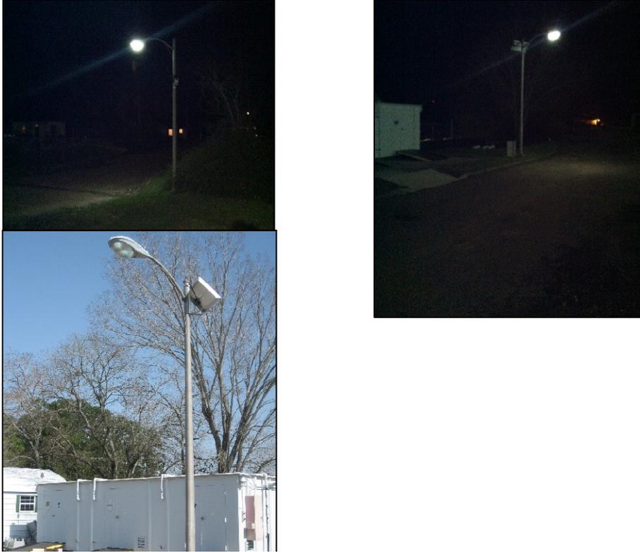
Figure 4. Retrofitted light pole housing, battery and controller boxes, LED light fixtures
